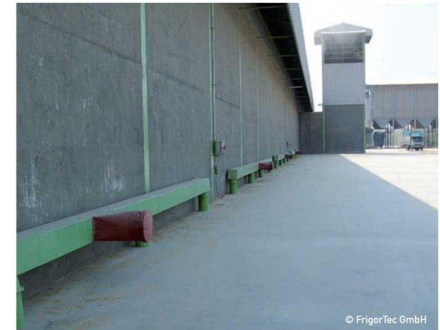
2 Warehouse storage with central air distribution for GRANIFRIGOR™ - grain cooling
